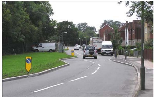
Recently a traffic calming scheme was introduced into the Magpie Hall Lane area (near Bromley Common). This includes a wide-area 20 mph zone, kerb build-outs and other measures. At the southern end of Magpie Hall Lane itself, where a new school is being built, this has resulted in a “chicane” like arrangement being built as shown in the photograph above.
