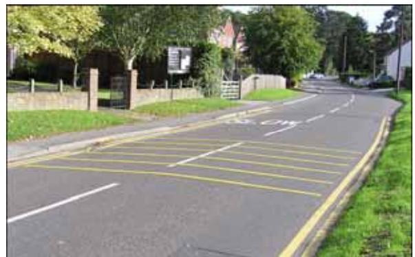
Above is a picture of a new traffic calming measure on Rushmore Hill, in the quaintly named village of Pratts Bottom. It consists of five sets of "rumble strips". This is road with a 30 mph speed limit, but on which traffic often exceeds that limit.
