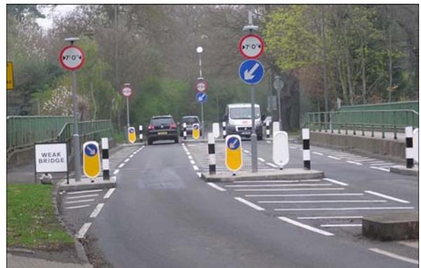
Many delays have been occurring on the railway bridge on Chislehurst Road (the road between Chislehurst and Petts Wood). A weight limit had to be imposed after an assessment indicated it could not support more than 7.5 Tonnes. This meant that one-way working was put in place temporarily but that has now been replaced by the width restrictions shown in the above photo.
